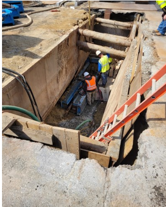
Pipe Bursting on Middlesex Turnpike
