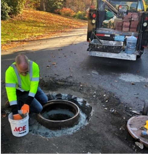
Adjusting Roadway Structures
