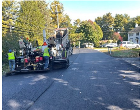
Asphalt Paving
