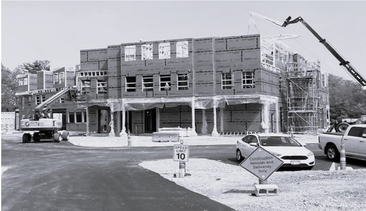
LCB Assisted Living facility under construction at 240-244 South Road
