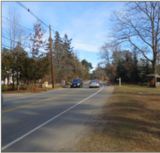
Existing condition: Lack of bicycle and pedestrian facilities on Concord Road
