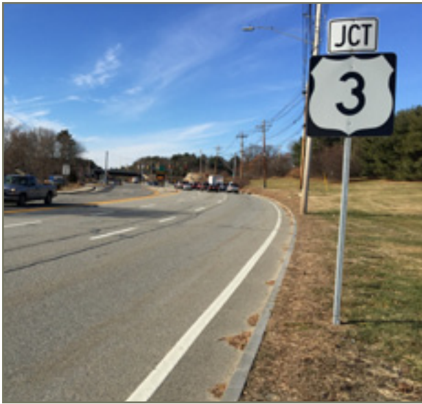
Existing condition: Lack of bicycle and pedestrian facilities on Burlington Road
