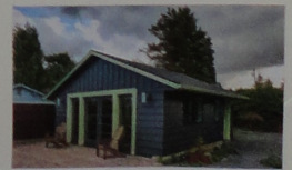
Detached unit in Estacada, Oregon Image: City of Estacada website
