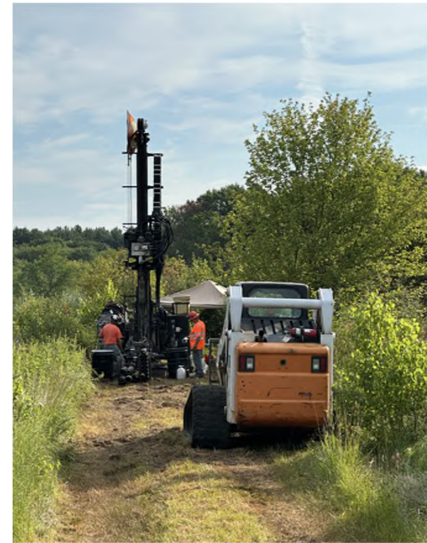
Soil boring being advanced.
