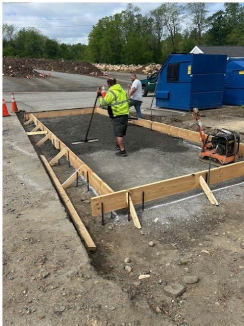
Compactor Foundation Construction
