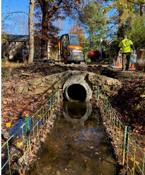
Glen Terrace Drainage Repair
