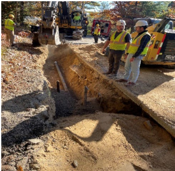
Water Line Replacement
