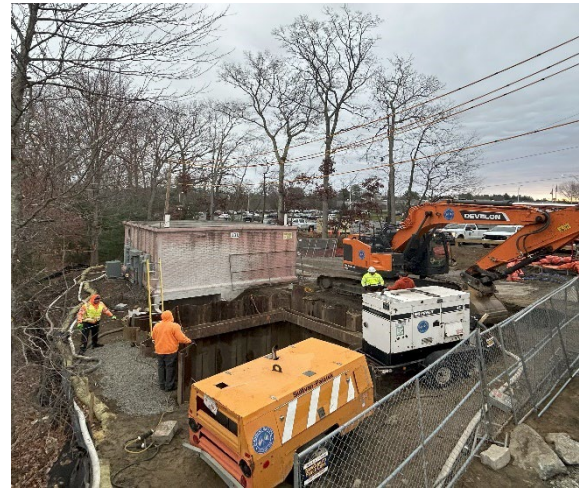
Middlesex Turnpike Pump Station Reconstruction
