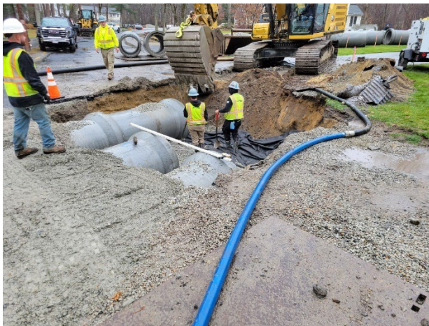
Richard Road Culvert Replacement
