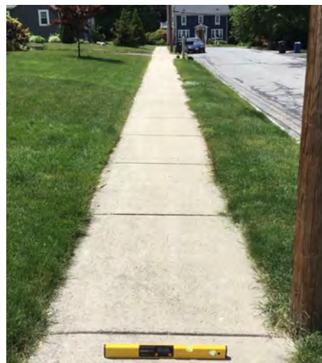
Fitchdale Avenue SCI: 86- Good Condition
