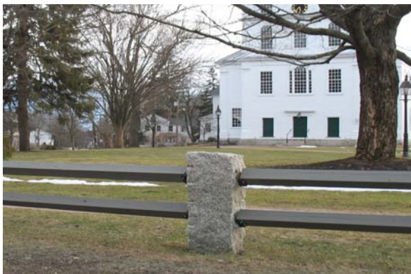
Double split-rail fence, with granite posts.
